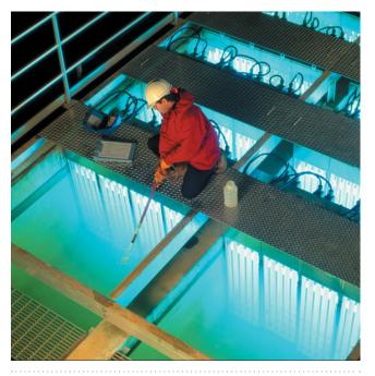
FIGURE 12.16 Ultraviolet light irradiates a thin layer of water, killing harmful organisms. (Flip Chalfant/The Image Bank/Getty)
