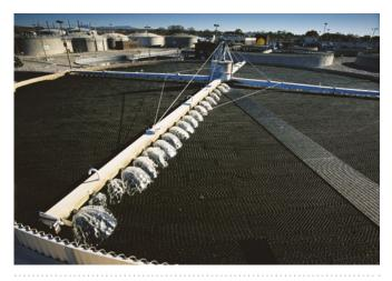
FIGURE 25.24 Trickling filters. These filters are used in secondary sewage treatment. (Jonathan A. Meyers/Photo Researchers, Inc.)
